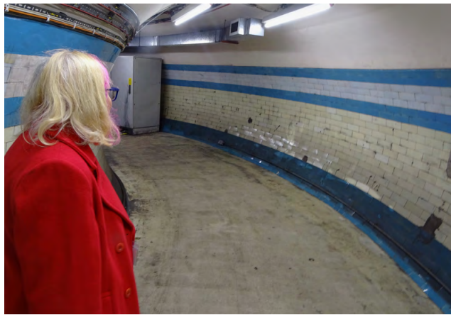
Empty Tunnels at Baker Street Station
